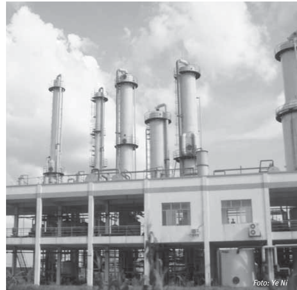
Moderne ABE-Fermentationsanlage in Guangxi China
